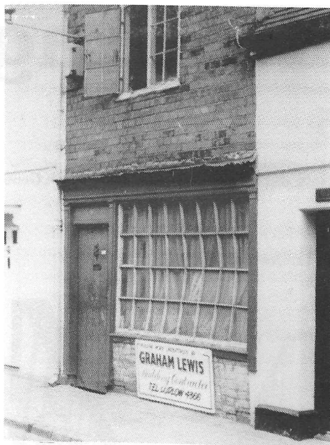
No. 16 Bell Lane: early nineteenth century shopfront
