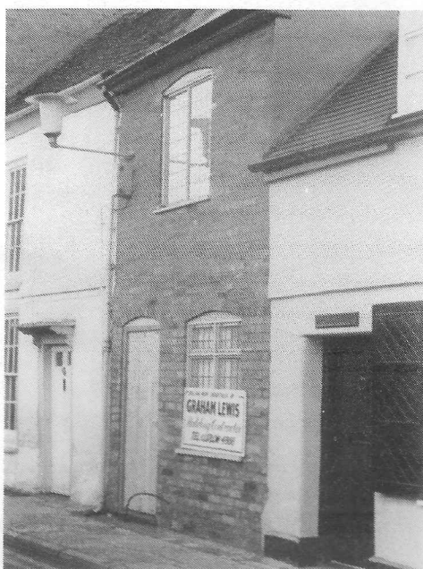
No. 16 Bell Lane: after alterations
