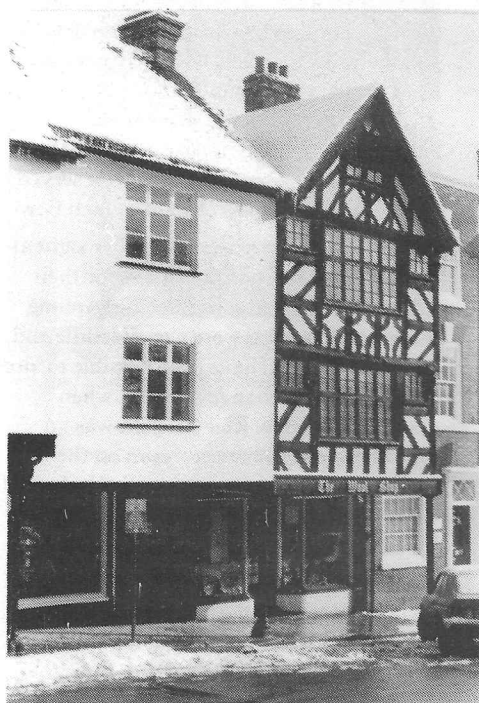
No. 10 Broad Street: the plaster work concealed a timber frame matching that of the neighbouring Wool Shop
