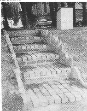
Steps down to the 'Dig'
