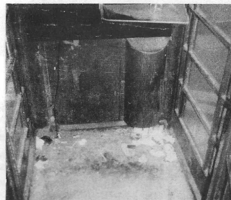
Litter on floor of Ludlow telephone kiosk
