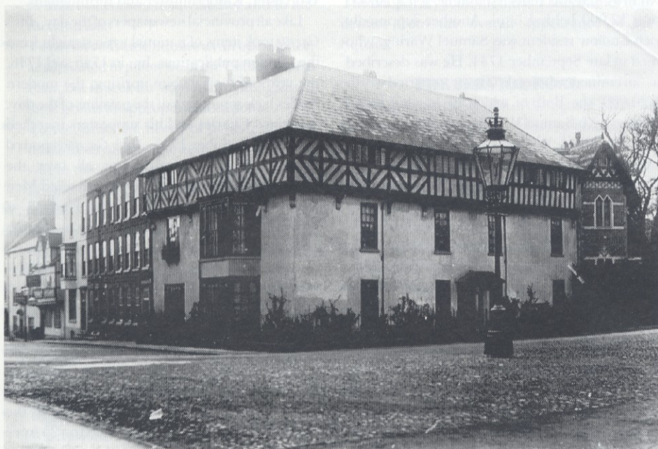
This detail from an early 20th century photograph shows Nos. 54-56 Mill Street. No. 54 (far left) had already been much altered by the insertion of a projecting bay and the removal of two windows from the second storey but Nos. 55 and 56 retain most of their original features.
