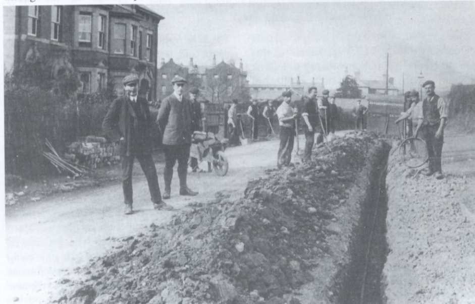
Workmen installing the electricity cable in Gravel Hill (Photograph courtesy of David Lloyd)
