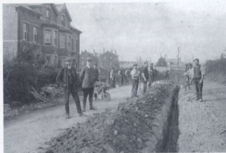
Laying the electricity cable at Gravel Hill, with the workhouse in the background (1908)
