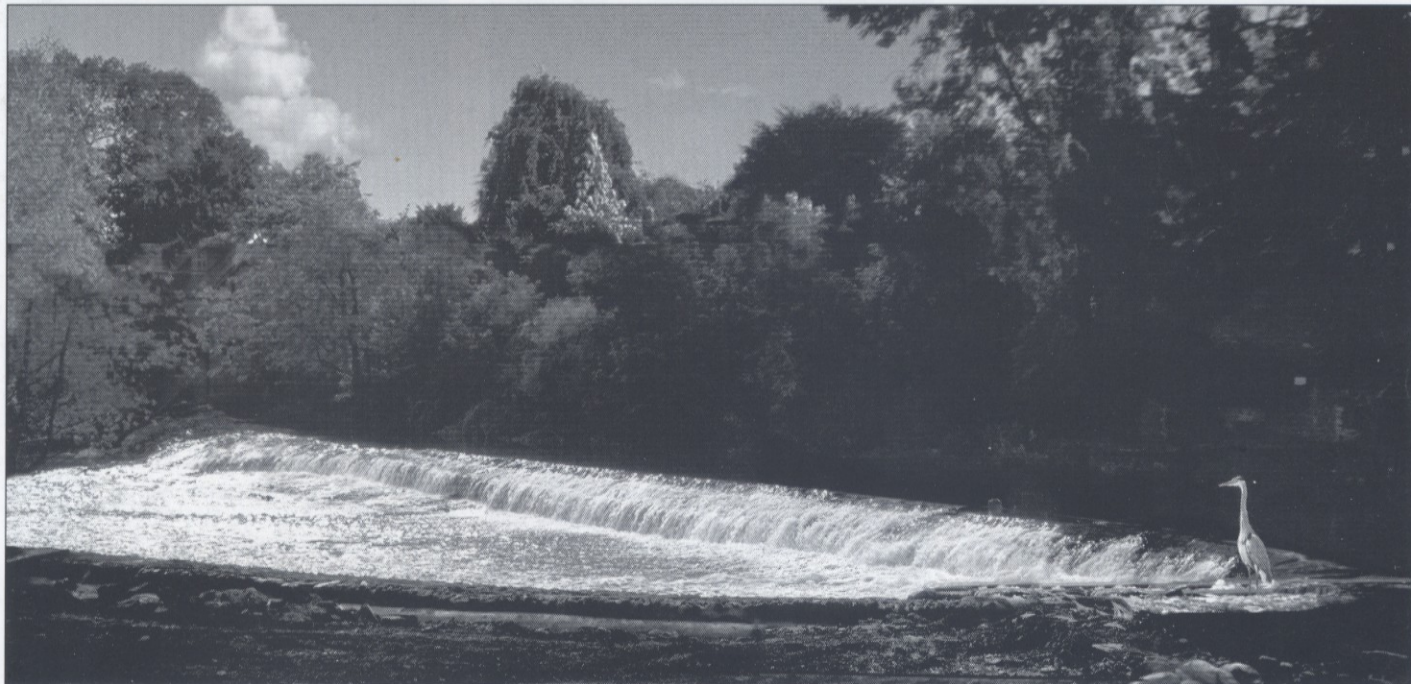
The restored Horseshoe Weir, with heron, at Ludford Bridge. We congratulate the Ludlow Weirs Trust on the completion of this project, to which the Civic Society gave its full support. Photo: Gareth B. Thomas F.R.P.S.
