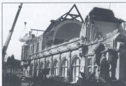
The demolition of the Town Hall in 1986.
