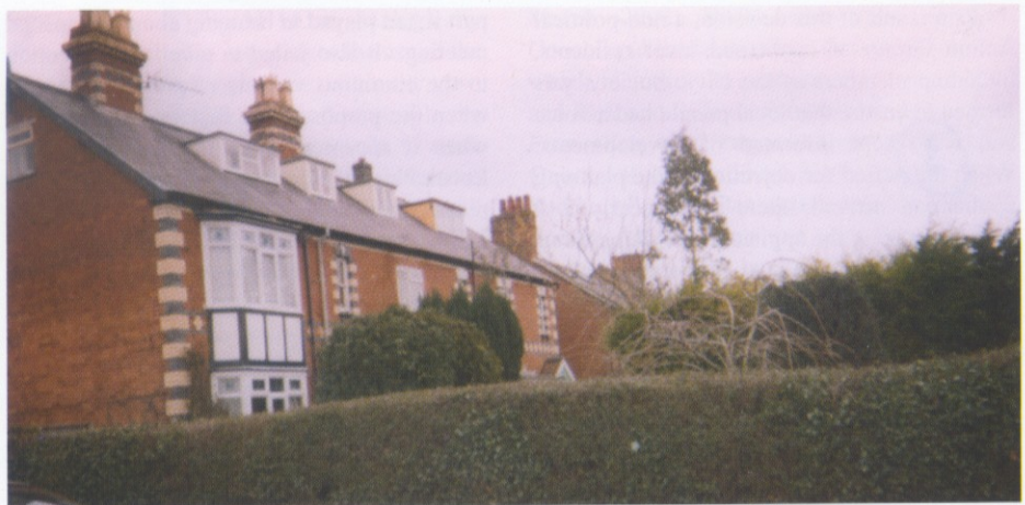
Julian Terrace, now backing on to Sandpits Road.
