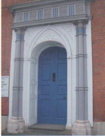
The doorway at the Guildhall, once at risk
