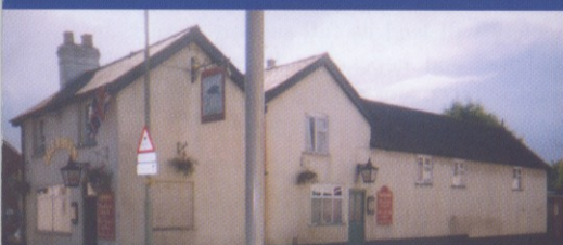
The Raven, to be demolished
