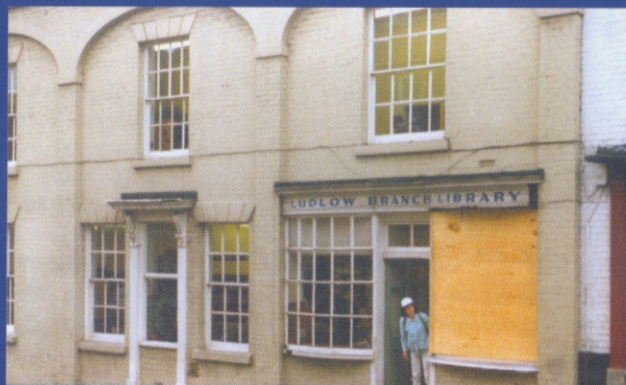
The old library in Old Street with its demolished window, later replaced
