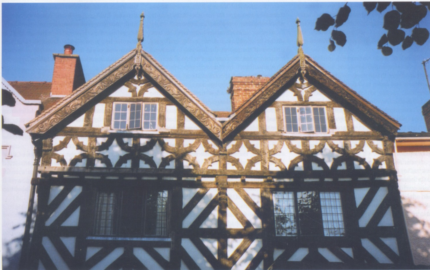
New and old. The restored bargeboards next to the originals.
