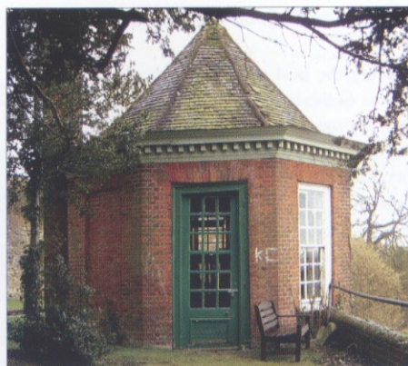
The Gazebo at Ludlow College
