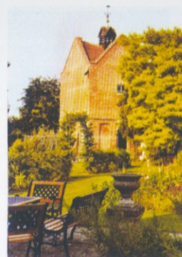
Fig 4. Georgian dovecote, Eardisland
