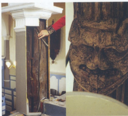
Left: A timber post inside its 18th century cladding Right: The grotesque head
