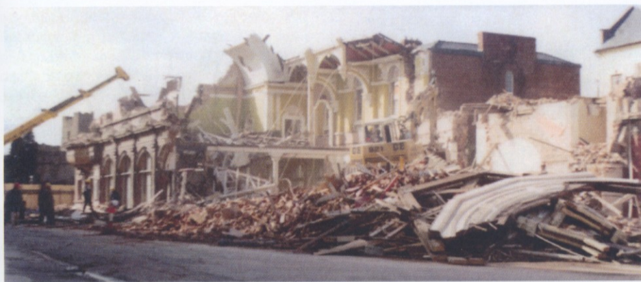
Above: Nearing the end - March 1986 Below: An early side view of the Town Hall. Opposite: The view from the Castle
