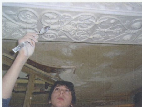
3. Putting final touches to the finished stamped position.
