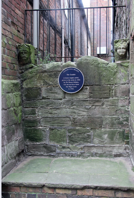
Fig.1 Water conduit Church Street Ludlow.
