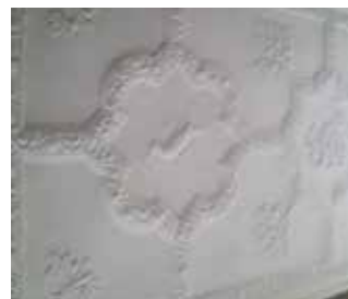
2. A section of the replastered ceiling in the drawing room.
