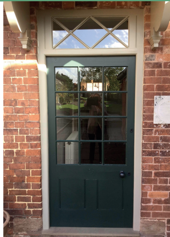
4. The reinstated fanlight
