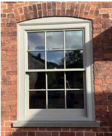
5. Replacement window sill using Forest of Dean stone
