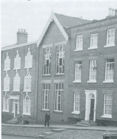
The 'Ballroom' in Broad Street, before re-fronting
